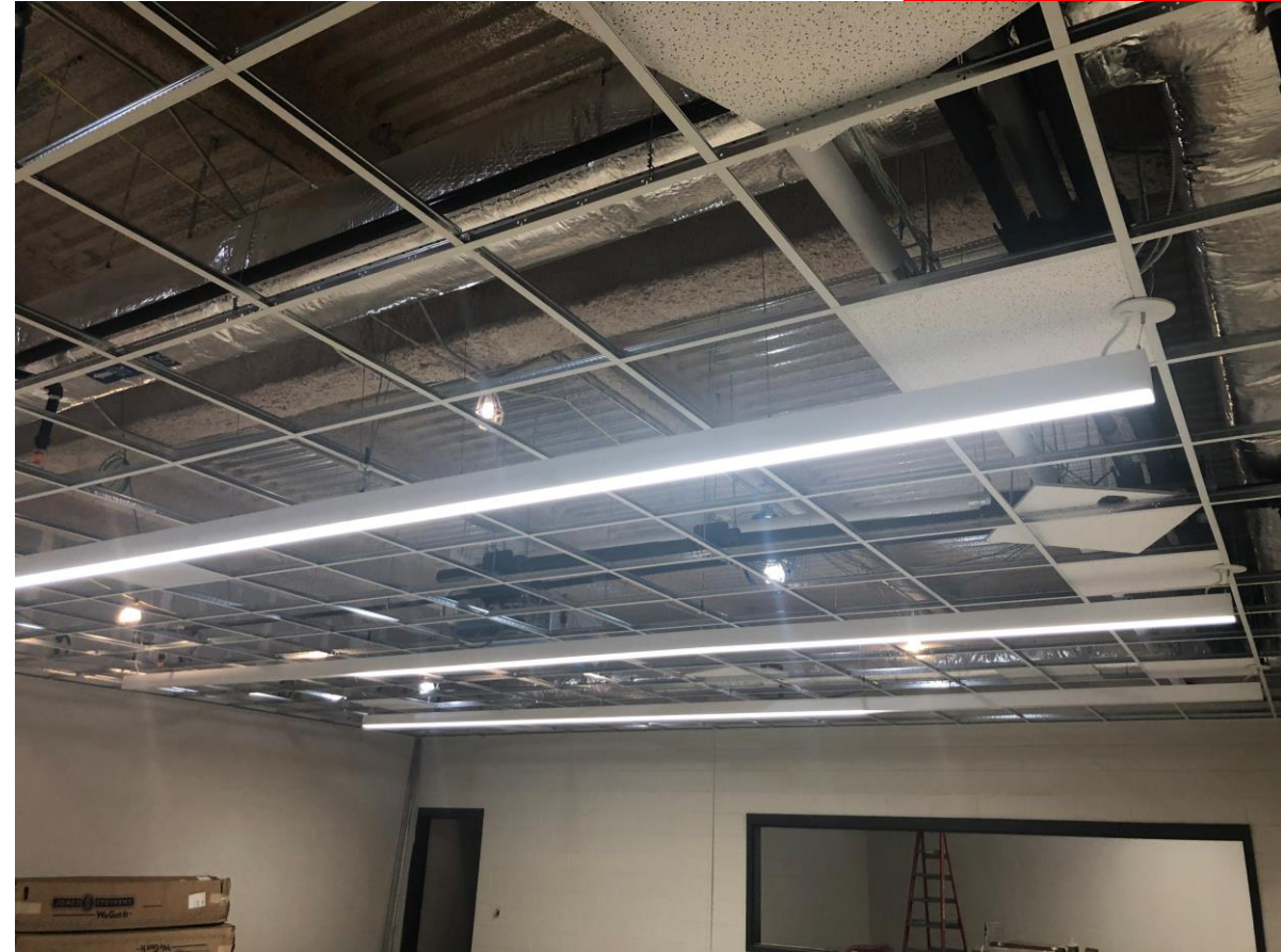
Light Fixtures Installed in New Addition Classrooms
